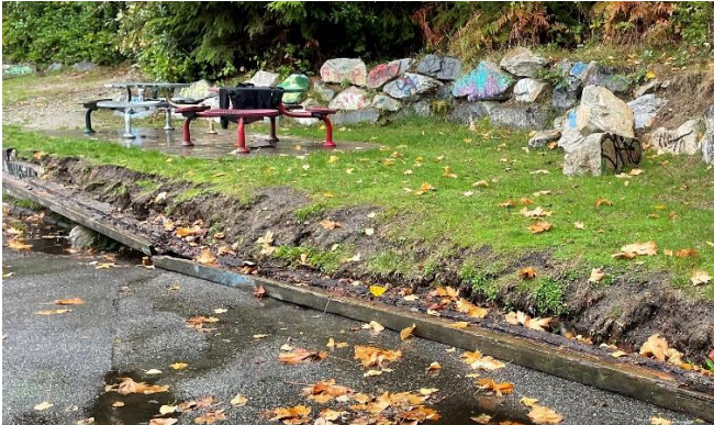
SKATE PARK BEFORE: Damaged rock and wood retaining walls
