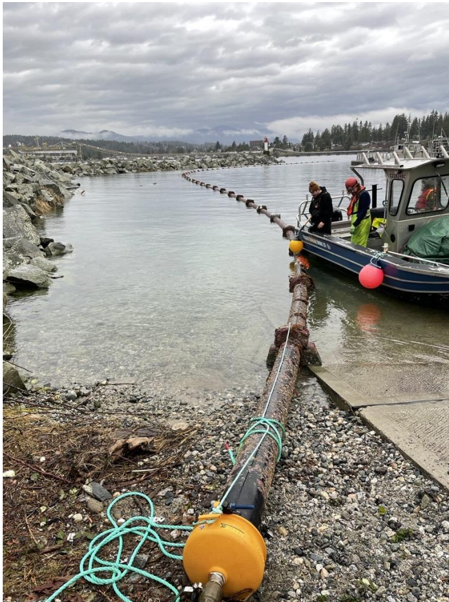
Launching effluent outfall pipe into Trail Bay
