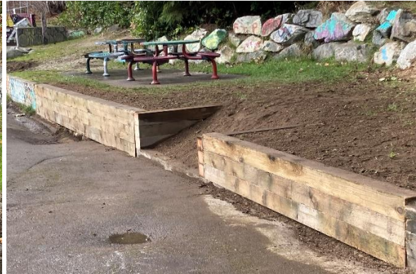
SKATE PARK AFTER: Rebuilt retaining walls and added ramp access to seating area
